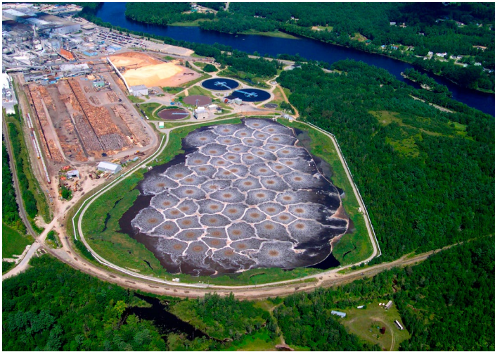
Verso wastewater lagoon, several round secondary treatment tanks and then off to get de-foamed before discharge into the Androscoggin. Photo: Point of View Helicopter Services
