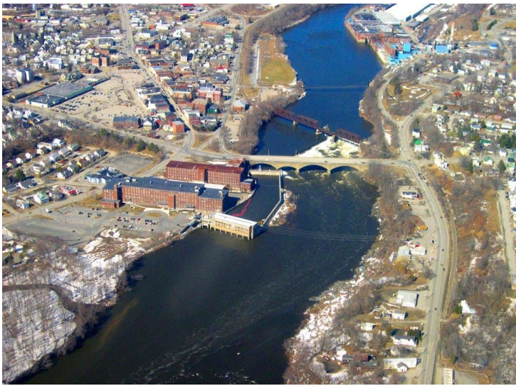
Lockwood Dam in Waterville, new “first wall” on the Kennebec. The dam is between the bridges. Fish passage and trap are at far left of the lower power house/turbine structure. Because fish move upstream in response to flows, most move into the 1/4 mile section below the dam. Only a few find the meager attraction flow from the fishway downstream. Photo: Point of View Helicopter Services.
